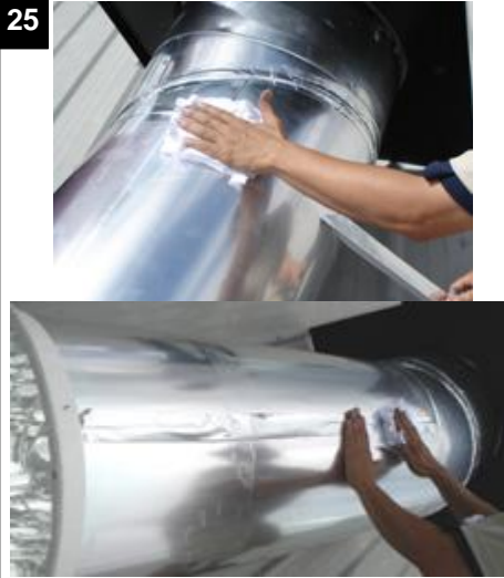
Use a cloth whilst applying pressure to the foil tape to ensure strong adhesion.
