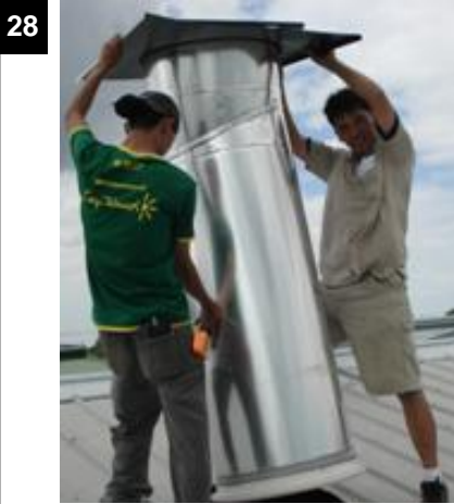
Now that the whole assembly is ready, insert it to the roof.
