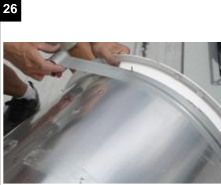
Put duct tape around the joint of the Ceiling Frame and the tube.
