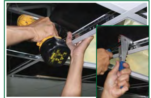
Step 6 - From the outside drill & rivet the Conversion Box Transition Piece to the Conversion Box Frame on 2 opposite sides.
