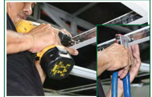
Step 3 - From the outside drill & rivet the Conversion Box Frame to the upright of the ceiling grid on 2 opposite sides.
